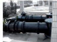
Pumping station II
