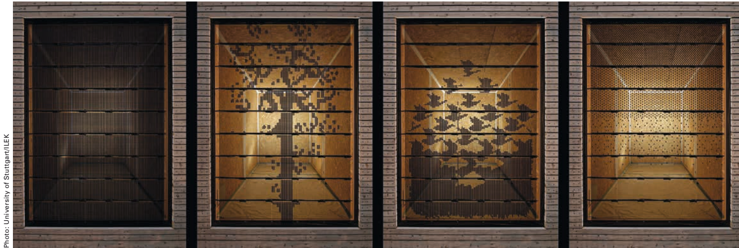
Switchable, pixelated glazing with various dimout factors and with different motifs.
