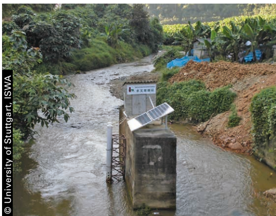
A water monitoring station in the catchment area of a Mekong tributary.
